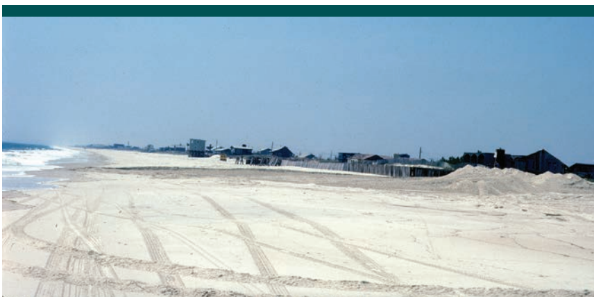
Figure 31. Beach scraping projects remove a thin layer of sand from the beach berm and push it landward to form a mound. This redistribution of a relatively small amount of sand on the beach probably has minimal impact, either positive or negative, on coastal processes or protection of the upland.
