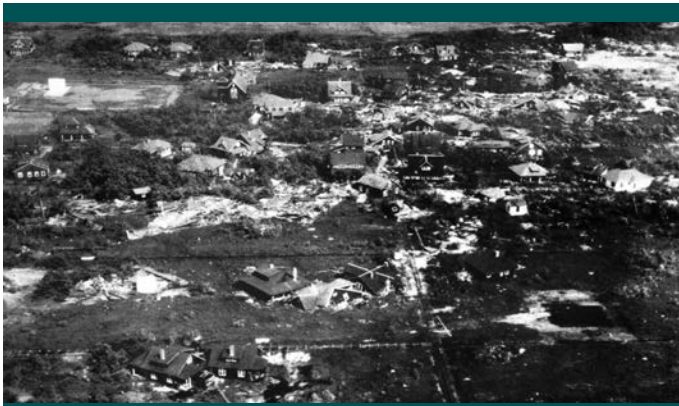
Figure 7. Damage in Saltaire, Fire Island, caused by the 1938 hurricane. (Photo: U.S. Army Corps of Engineers 1958)
