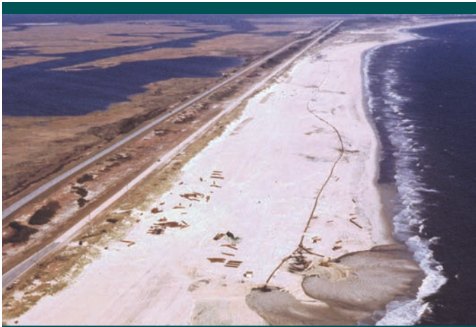
Figure 26. Inlet bypassing and beach nourishment project on Jones Beach Island. Sand dredged from Fire Island Inlet (in the background) is piped to the site and deposited on the shoreline to build a beach to protect the Ocean Parkway. (Photo: American Dredging Company)
