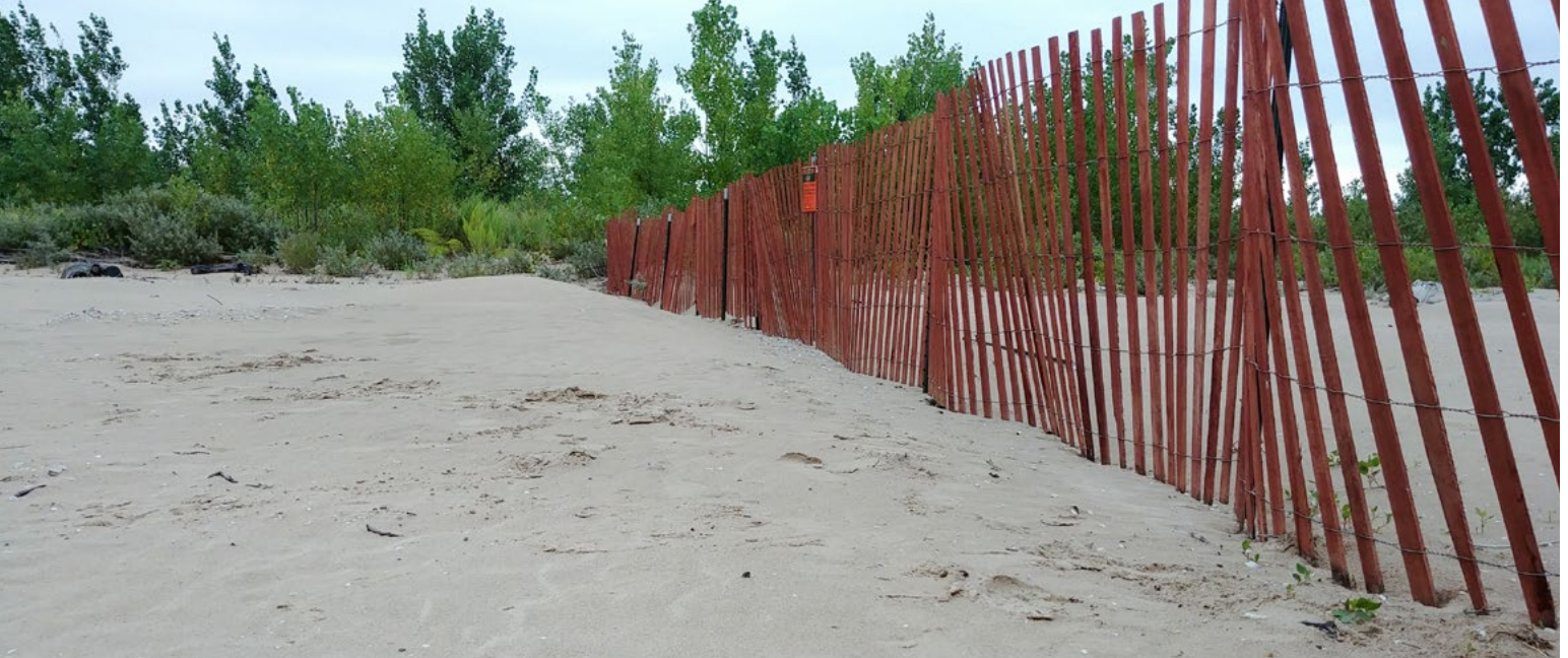
▲ Sand is deposited on the leeward (downwind) side of fencing on the Lake Ontario shoreline at Sandy Pond. Sand fencing contributes to the restoration of sandy beaches by trapping sand behind the fence line and allowing native vegetation to reestablish. Photo by Roy Widrig, New York Sea Grant.
