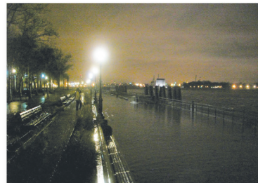
The promenade at the Battery was also completely inundated from the flooding event. The seawall is pictured here on the right.
