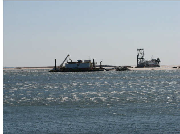
Dredging in Fire Island Inlet, New York. Photo: Jay Tanski, NYSG
